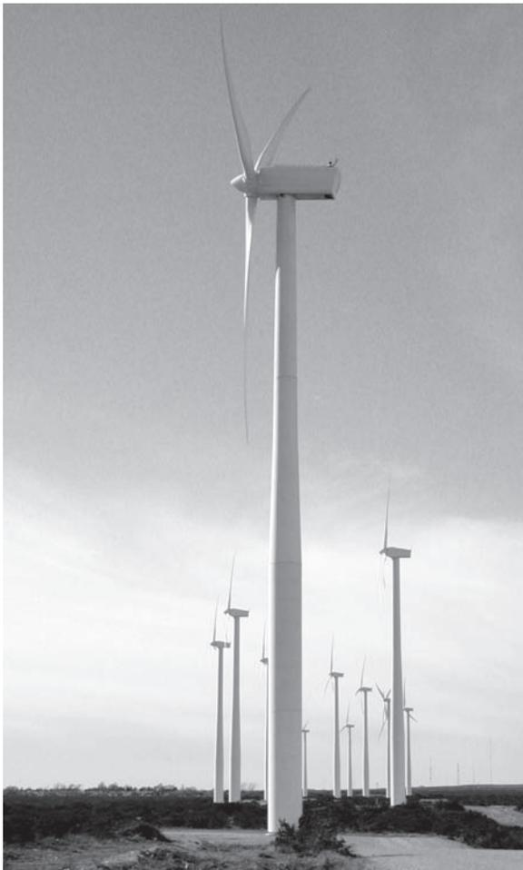
**LARGE MODERN WIND TURBINES** In foreground is the 1.65 MW wind turbine at Big Spring; in the background are 660 kW units.
